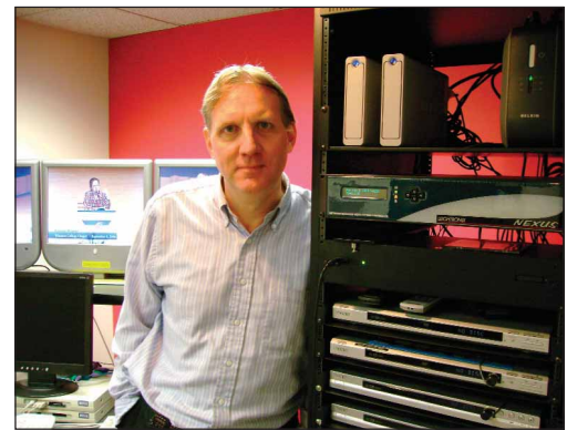
John Rorvik with Leightronix equipment installed at Wheaton College
